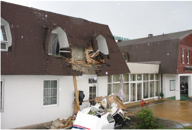
Tracks after the crash against the hotel building
